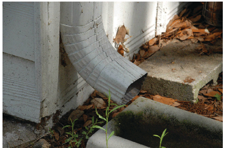
Figure 14. Gutter downspout—a possible colony nest site.
