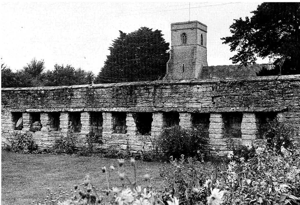
Figure 10. The hive recesses at Charity Farm, Lovington in Somerset, c.1953. IBRA Register, no. 131. Photo: Harold C. Tilzey. Cf. Figure 9.
