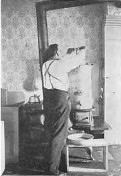
Fig. 108—Screwing Down Wax-Press.
