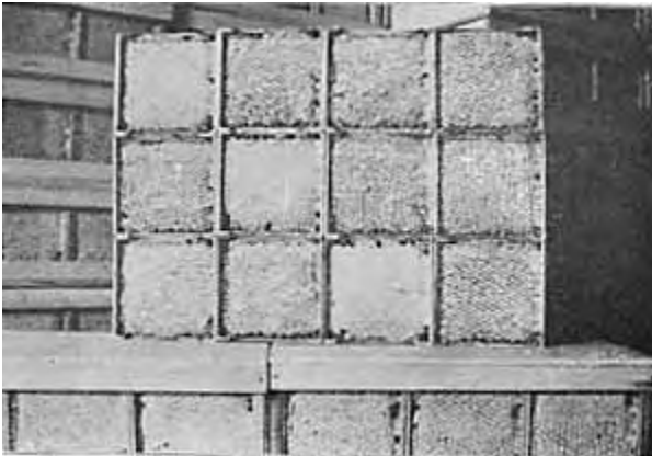
Fig. 100—Sections Ready for Casing.
