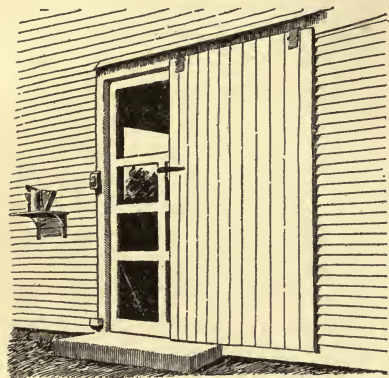
FIG. 18. — Honey-house door. The wooden door rolls clear of the opening and the screen door swings both ways.
