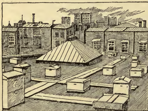
FIG. 15. — Roof apiary in lower New York City.
